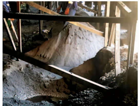
Spillage was pervasive, requiring regular cleanup which raised the cost of operation. © Martin Engineering 2024
