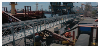
Full loading system — dual bay truck unloader with enclosed rear doors feeding a fully enclosed Telestacker conveyor into vessel.
