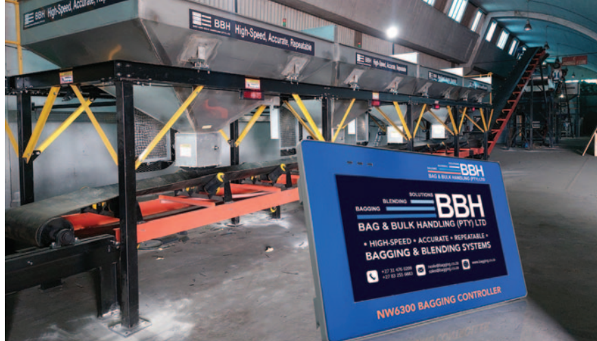
Batch blending system - Mozambique
