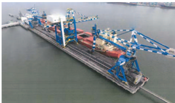
Detailed design of a new coal import conveying system for a power station in Malaysia included the upgrade of the existing grab-type ship-unloader (above, left) and adding a new conveying stream from the import jetty to the existing power station stockyard facility (above, right).
