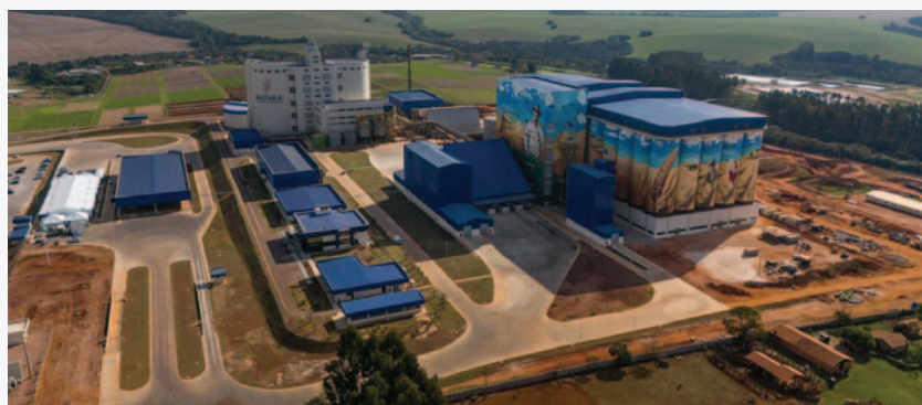
Cooperative Agrária Agroindustrial (Agrária) and co-operative partners — Bom Jesus, Capal, Castrolanda, Coopagícola and Frisia — recently celebrated the commissioning of Maltaria Campos Gerais, the largest malting plant in Latin America (photo: permission of Agrária).
