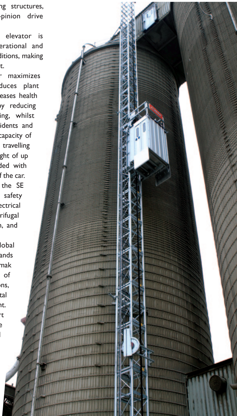
Alimak Group's SE 240L elevator, designed for installation on silos, storage vessels, cranes and other industrial applications, eliminates the need for a machine room or a supporting elevator shaft, reducing building requirements and ongoing structural maintenance.
