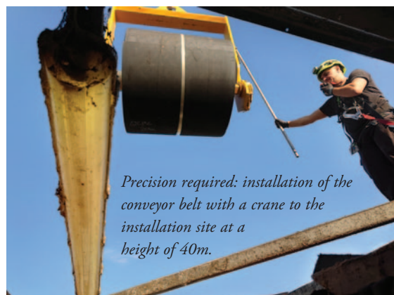
The REMA TIP TOP experts select a special conveyor belt profile for optimum material transport of the moist woodchippings.
