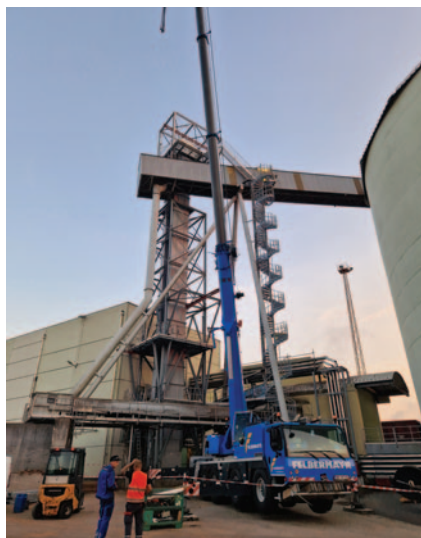
REMA TIP TOP installs the conveyor belts at a height of 40m at Lenzing.
