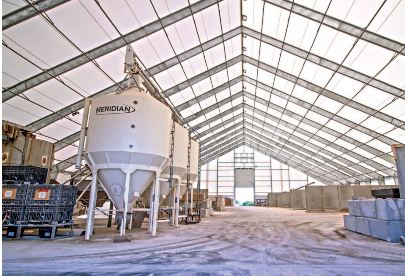
Legacy structural steel frame.
